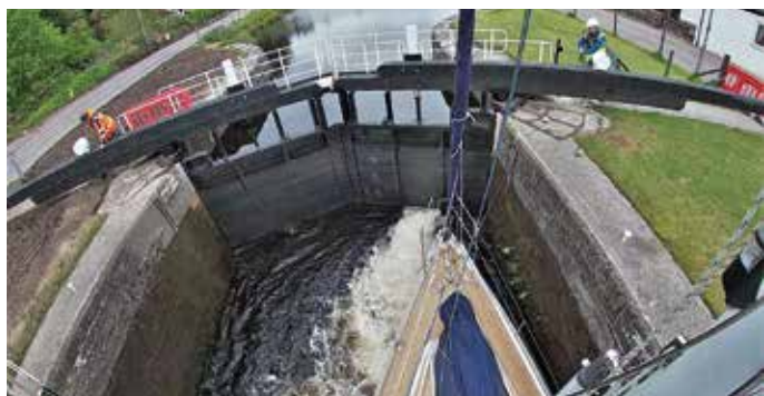
The sluice on the same side as the forward boat is opened first to keep the bow in
