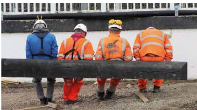
The hydraulic rams were not yet operational
